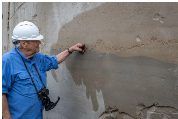
Inspecting some interesting structures; Bloomington 2019
