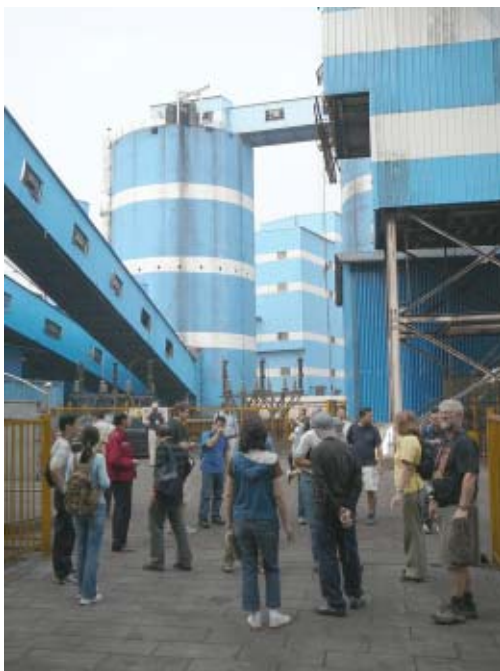
Pingshuo coal preparation plant. C Ward photo.
