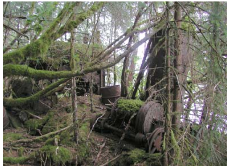
Figure 7. Boiler and winch near the mouth of the Kootznahoo Inlet coal mine. T. White photo.
