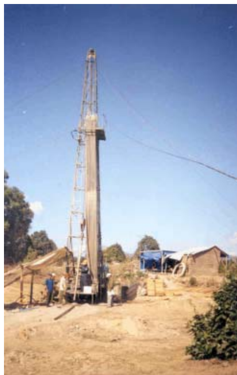
Fig. 3. (A) The drilling rig of Enreca-1
