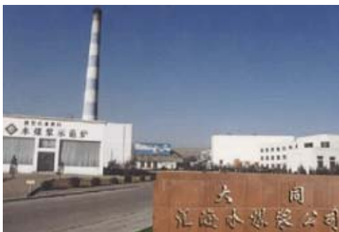
Datong Coal Slurry plant
